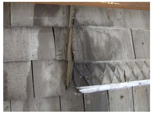
Image 3.5.15. The Gables, (Building B), west elevation, detail of 1923 building (left) abutting 1901 building (right), 2008. Christopher Pollock photo.
